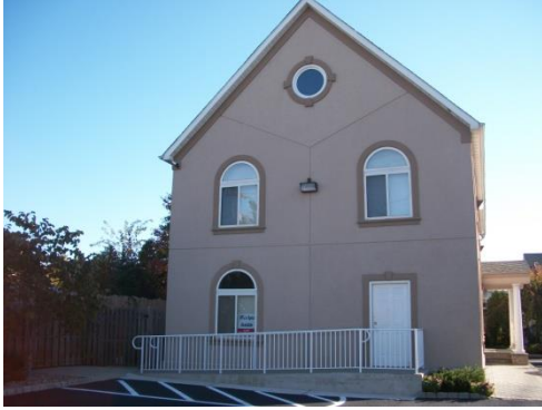
ADA Assessable Side Entrance
